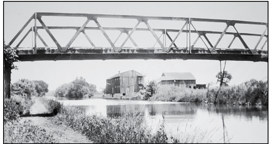
White's Ferry granary and warehouse.
