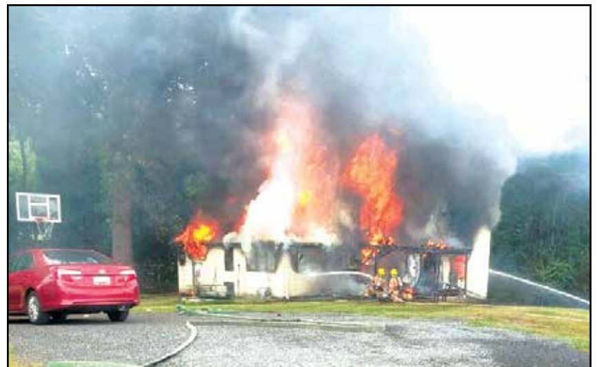
The fire department was met with a raging fire upon its arrival.
