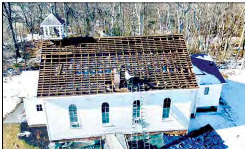
Sugarland's historic St. Paul's Church gets a new roof.
