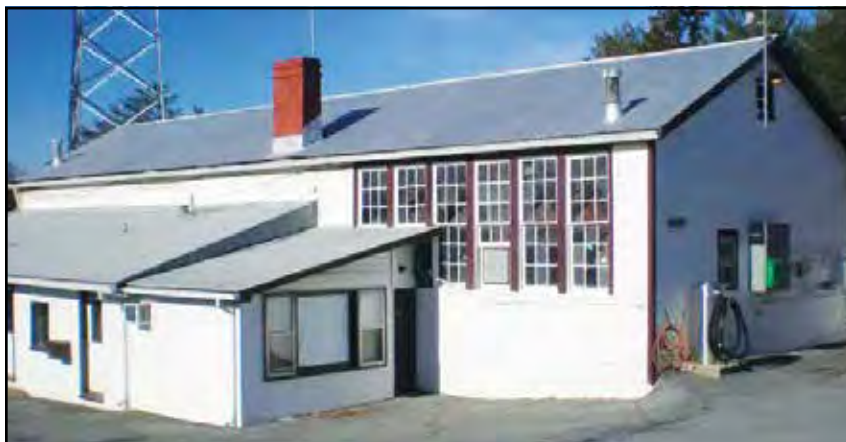
In 1917, the Rosenwald Fund donated more than $70 million for educational and cultural facilities nationwide. This one still standing at our local Beauty Spot was part of that program.
