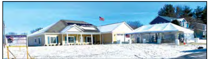
The Homes for Our Troops home for severely-injured post-2011 vet Manny Melendez-Diaz is at the corner of West Willard Road and Westerly Avenue.
