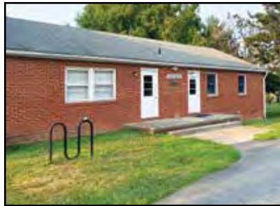
This former youth center at Poolesville Memorial United Methodist Church is being considered as a new site for WUMCO.
