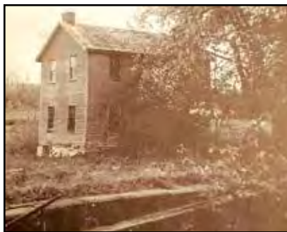
This photo of Lockhouse 26 was taken in 1948. The lockhouse burned down in 1969. More about the residents of the lockhouse in In Your Own Backyard on page 12.
