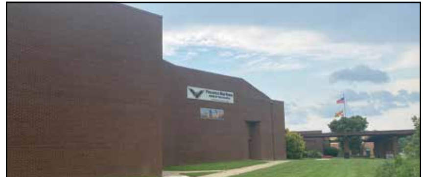
Under all design proposals for a new school, the auditorium will remain and will be refurbished.
