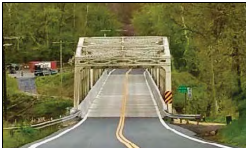
The long wait to complete the refurbishment of the Monocacy Bridge will hopefully come to an end on October 1.
