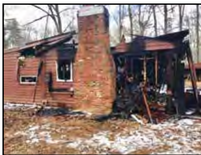
A fire on Budd Road destroyed this home. More on page 5.
