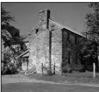
The original East Oaks Estate. Read about its history in Foundations on page 10.
