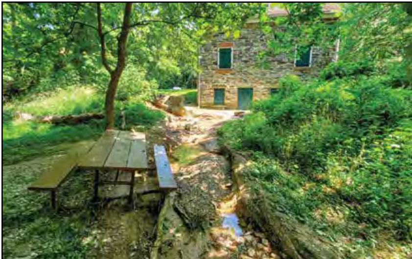
The torrential rains caused serious havoc to parts of the C&O Canal. Here, the picnic table was moved from the hill on the left, and a crevice was cut by the overflow of water from the canal.
