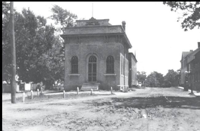
New sidewalks replaced the old wooden planking.
