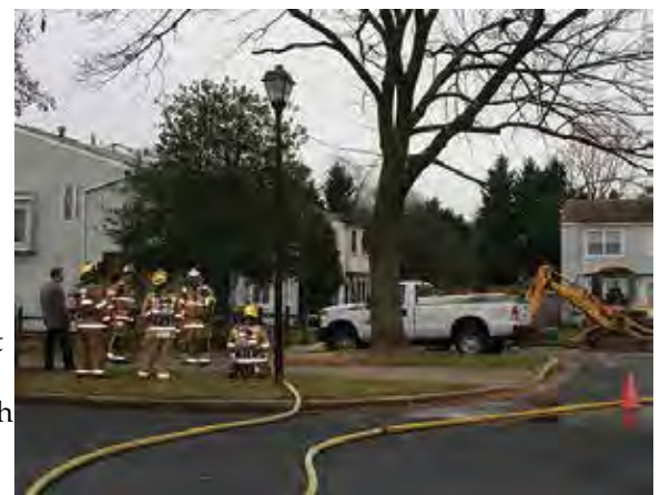
Town Manager Wade Yost and firefighters at the site of a recent gas leak.
