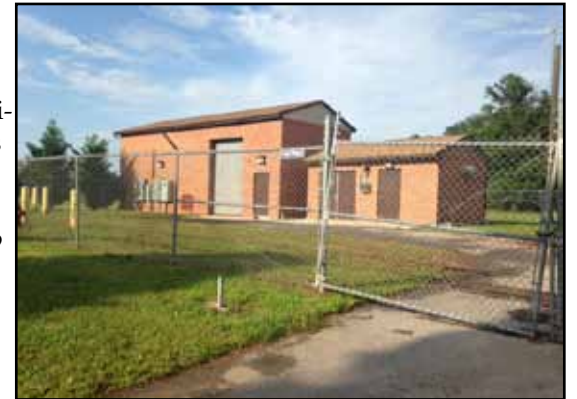
The pump house on Budd Road was the subject of a legal settlement.
