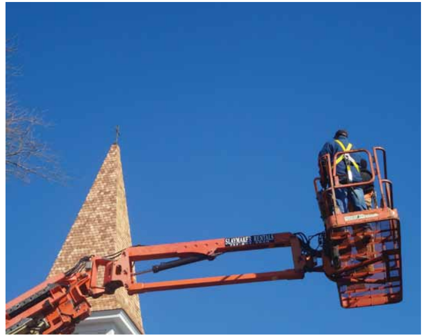
A strapped-in Ted Wroth rides up to inspect the steeple and new cross at St. Peter's.
