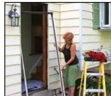
Marie Easterday inspects her damaged rear door.
