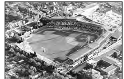
An undated photograph of Griffith Stadium, which stood at the corner of Georgia Avenue and W Street, NW, in Washington, D.C., the present day site of Howard University Hospital.
