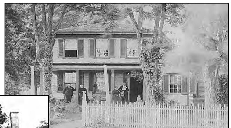
The Hall Home: Now the parking lot of M&T Bank.
