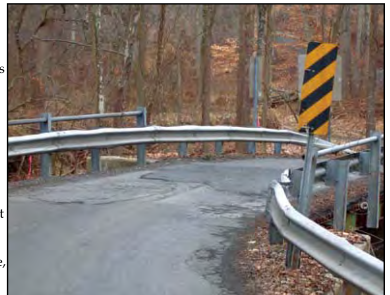
The bridge on White Ground Road.
