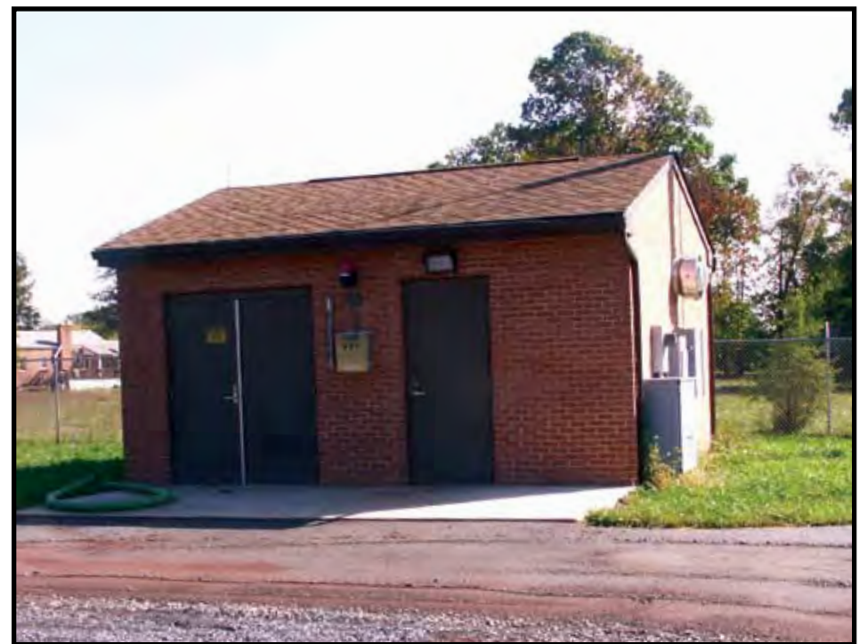
The well house for Town of Poolesville wells number nine and number ten.
