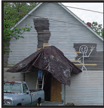
The Barnesville Town Hall under restoration.
