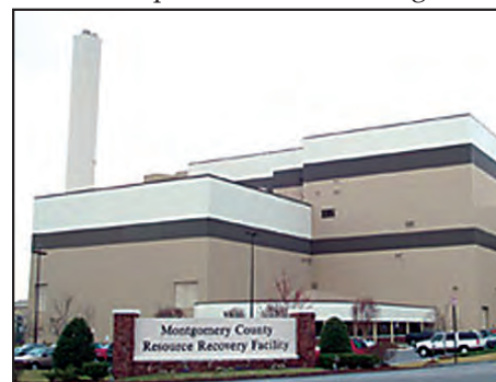
The Montgomery County Resource Recovery Facility, where the mercury was recovered.
