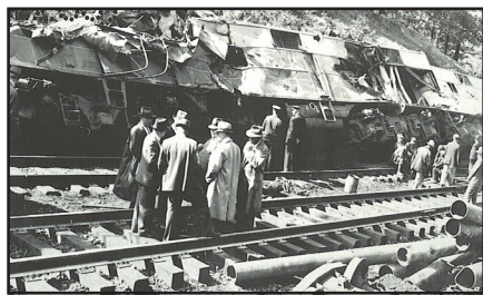
Historic train accident in Dickerson.
