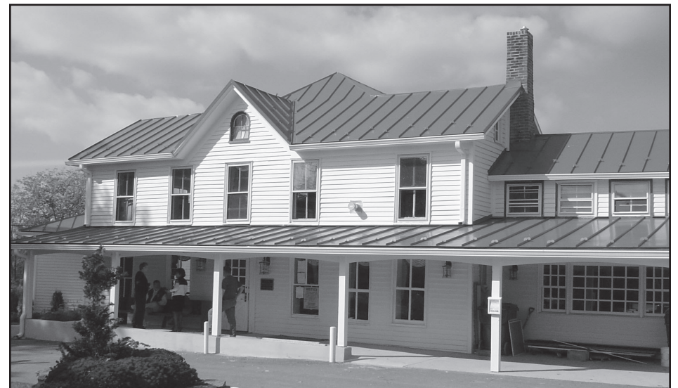
The almost-finished Comus Inn at Sugarloaf Mountain.
