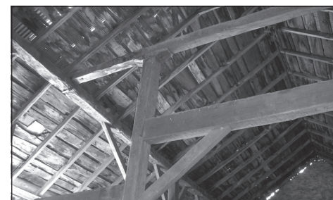
Hand-hewn beams have held the barn secure for 165 years.
