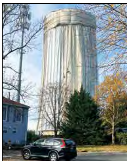
Poolesville's water tower is undergoing a facelift.
