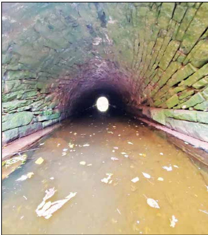
Culvert 65 of the C&O Canal: the "1832" culvert.
