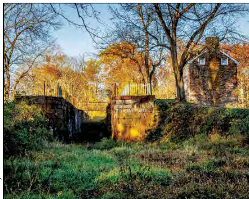
Here, the Seneca Aqueduct and Lock 24 are combined into a single structure. The only place along the canal where this was necessary. The aqueduct and lock are made of Seneca red sandstone quarried just west of here. That same sandstone was used to build the Smithsonian Castle in Washington, D.C. Construction of the aqueduct and lock was completed in 1832 at a cost of $32,000. Lock 24 is also known as Riley's Lock.
