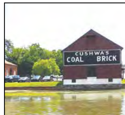
The Cushwa Brick building, the headquarters for the C&O Canal National Historical Park in Williamsport, Maryland
