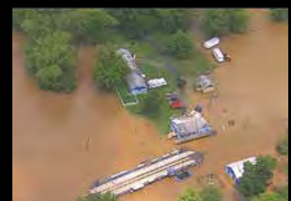
White's Ferry is prone to flooding given its location on the Potomac River. Aerial photographs show the extent of the flooding.
