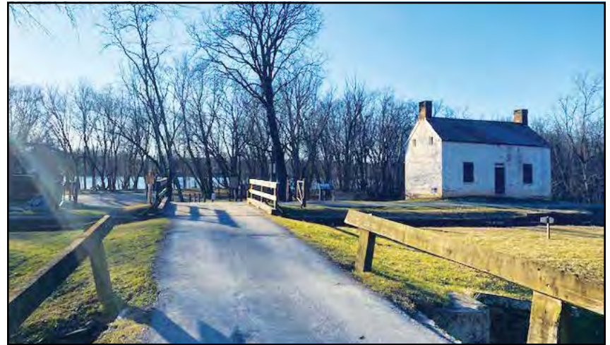
Edwards Ferry boat ramp is now inaccessible due to the closing of the bridge.
