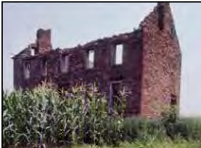
The ruins of the Richard Dawson home. Read about it in Foundations on page 4.
