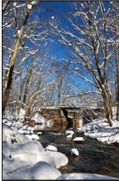
The Broad Run Trunk Aqueduct spanning Broad Run.
