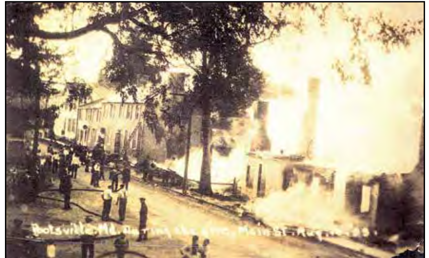
This August 16, 1923 fire started in the building that predates the current Williams Store next to Poolesville Tire and Auto.
