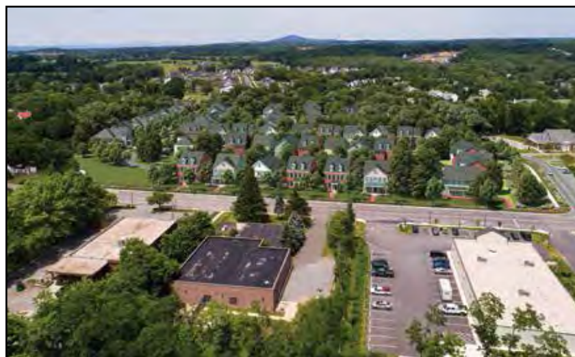
An aerial virtual reality picture of the proposed Willshire Community looking north.
