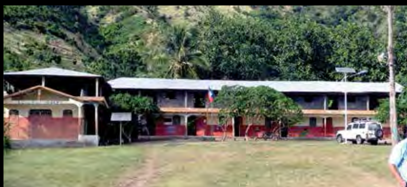
Before and after photos of the decimated school in Carcasse after Hurricane Matthew's devastation. Bottom photo shows the complete destruction of the village's church.
