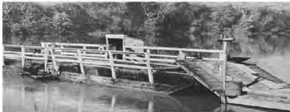
This is one of the earliest pictures of White's Ferry as a powered ferryboat. Prior to that, boatmen used poles to push it across the Potomac River.
