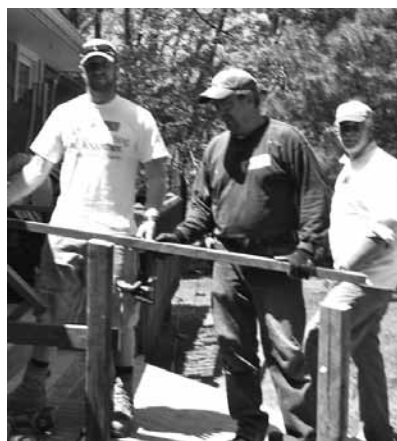
This Rebuilding Together Team made up of Connor Kraegel, Steve Kocur, and Bill Kraegel placed a handicap rail leading to the home.
