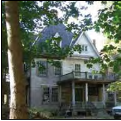
The owners of this house earned their wealth by inventing the sowing bobbin. Learn more in Foundations on page 15.
