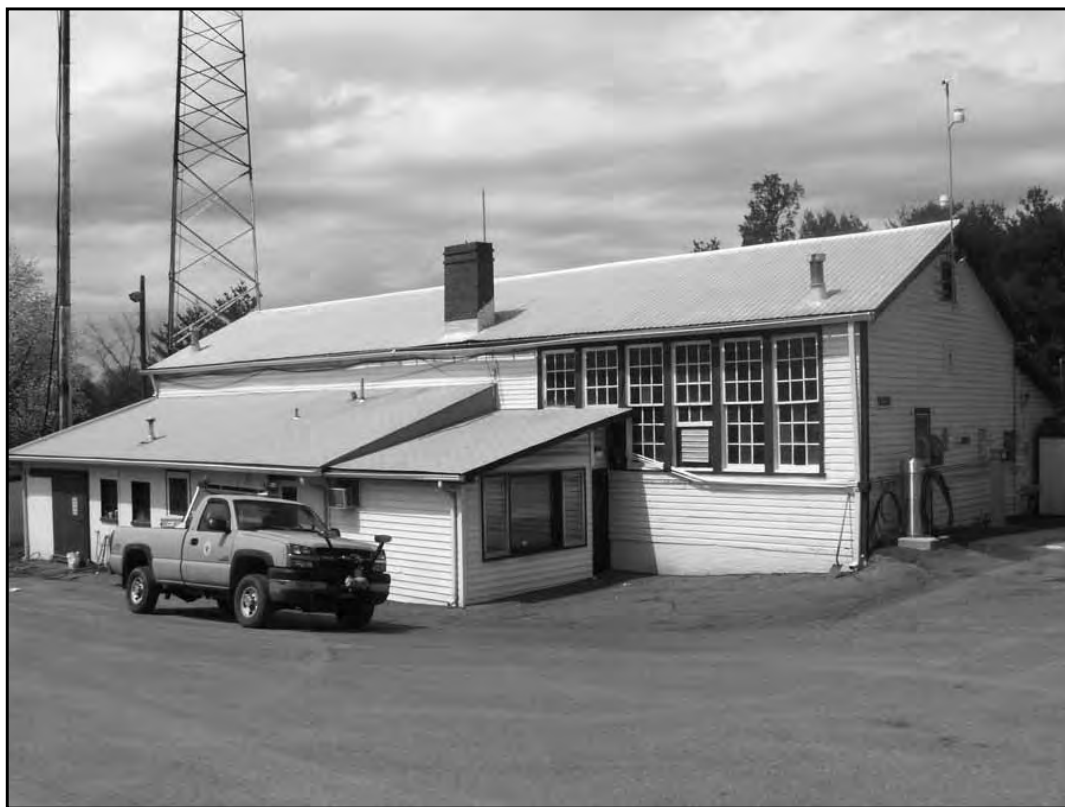
This building on Jerusalem Road in Poolesville is recognized by many as the offices for the Upcounty Beauty Spot. Are you aware of its special role in county education history?
