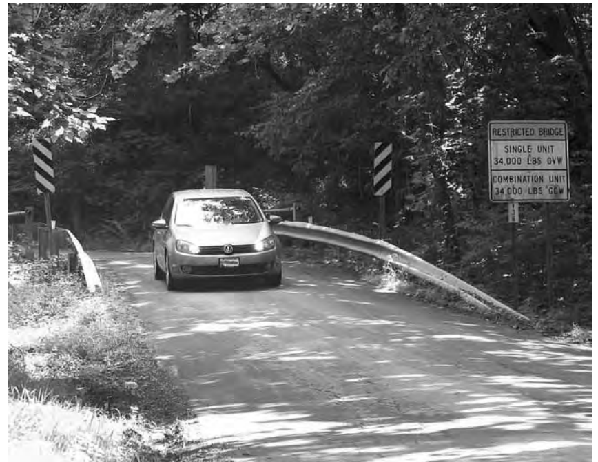
White Ground Road over Seneca Creek
