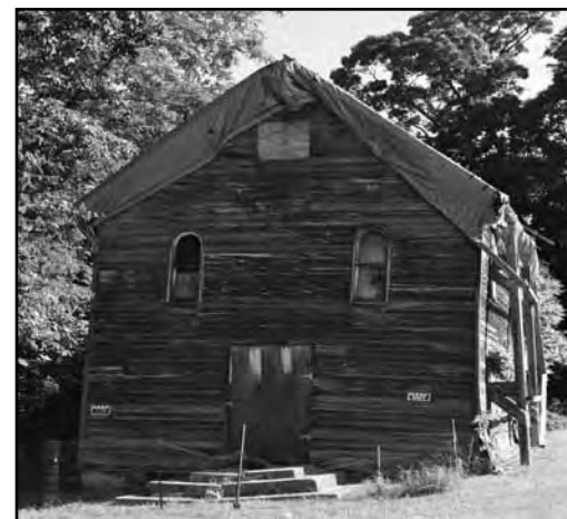
Charity Hall is scheduled for renovation.
