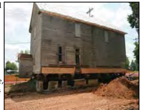
The Old Darby Store in Beallsville is about to move twenty-seven feet.
