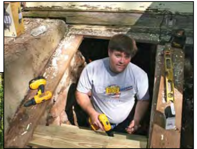
Eddie Schwartzbeck replaces a defective stairway to the basement.
