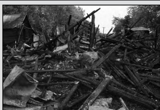
A fire broke out at last Saturday at midnight at the abandoned house on the north side Route 107 near Partnership Road. As an abandoned home, the fire department monitored the burn to prevent it from spreading. The cause of the fire has not been determined.
