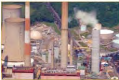
Chalk Point Generating Station
