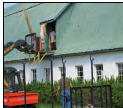
Workers put the final touches on the MOOseum
