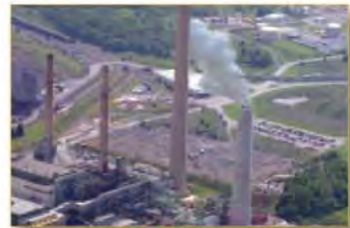
Dickerson Generating Station
