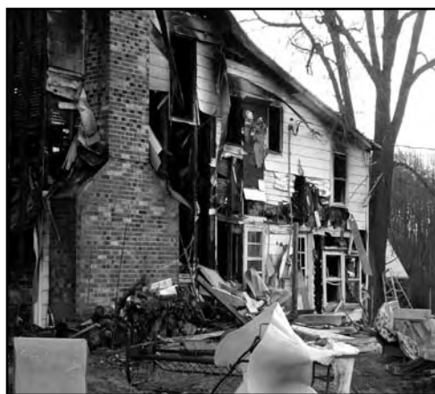
The remains of the Barnesville house that burned.
