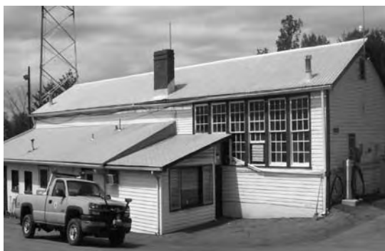
This building on Jerusalem Road in Poolesville is recognized by many as the offices for the upcounty beauty spot. Are you aware of its special role in county education history?
