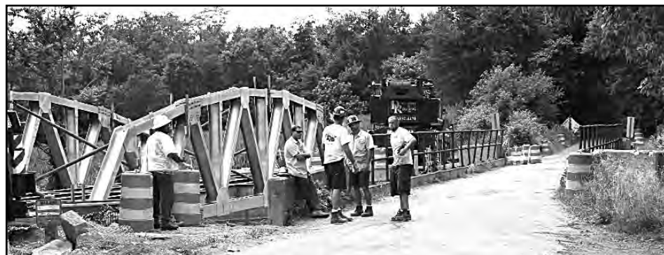
The new bridge, ready to replace the old bridge.
