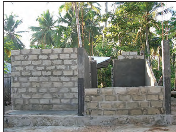
The building in progress.
