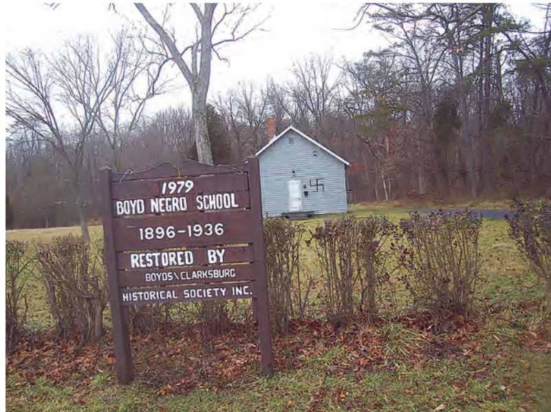
The vandalized Boyds Negro School.
